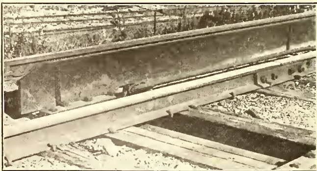
THIRD-RAIL PROTECTED BY BOARD AT THE SIDE
